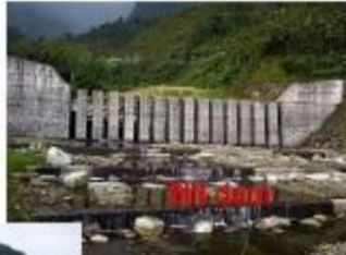
Ground sills established in riverbank
