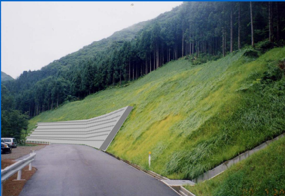
Retaining Wall (Image)
