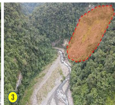
凹岸冲刷，崩塌淤積河床
