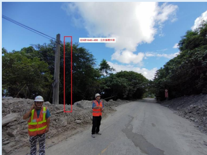
災後立桿點位現勘
