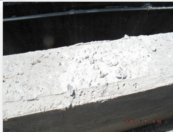
擋土牆澆置後未鏟平不平整
