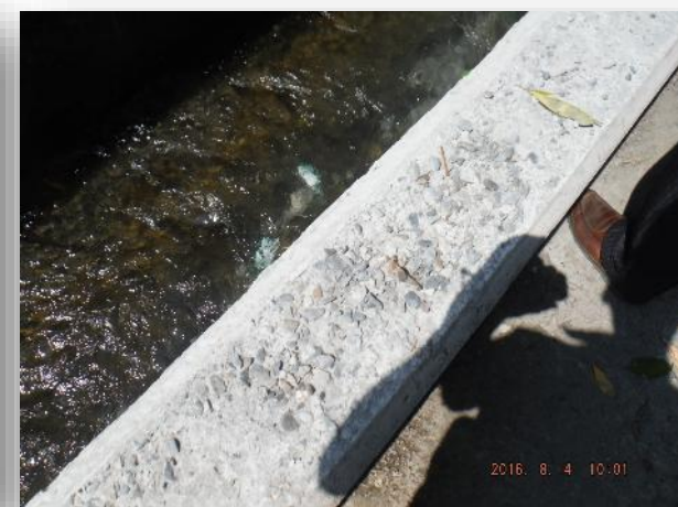
擋土牆澆置後未鏟平不平整
