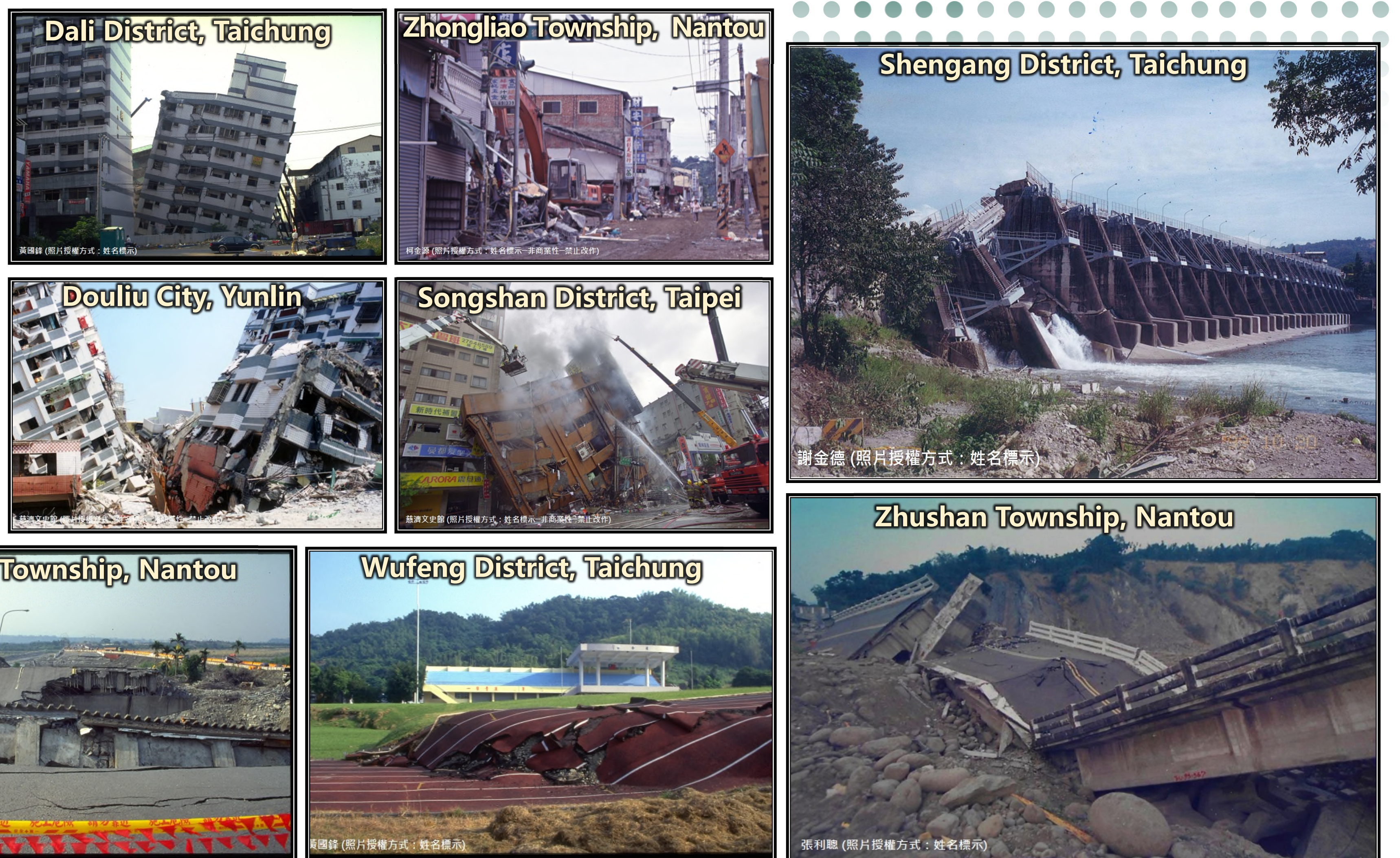
This disaster event resulted in over 2,400 deaths, more than 10,000 injuries, and nearly 150,000 houses partially or completely collapsed.
