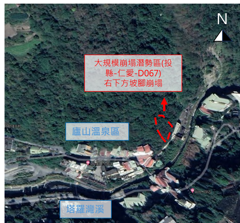
災害前遙測影像 (20221226_google earth)
