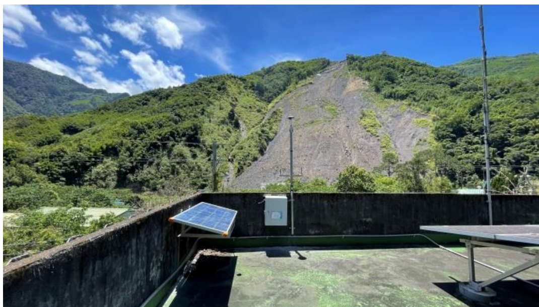
圖 4-11 LoRa-GNSS+GNSS-RTK Base (GW)
