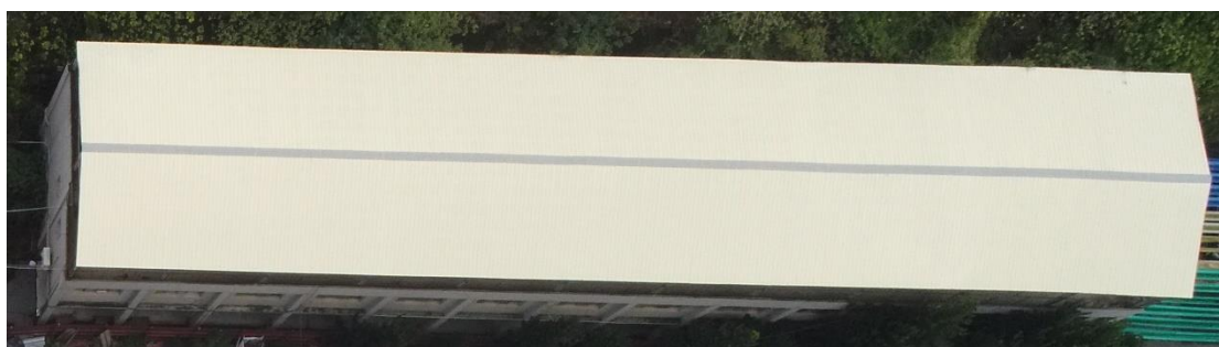
(b)P02 滯洪沉砂池
