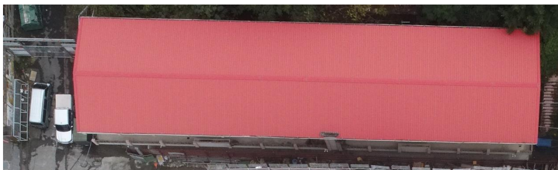
(a)P01 滯洪沉砂池
