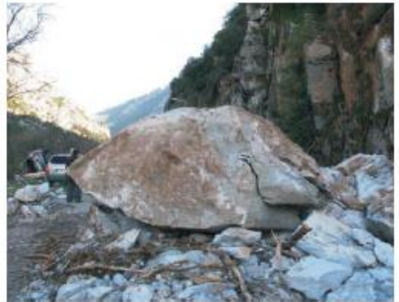
Figure 27. Severe rockfall along an expressway; cars were crushed
