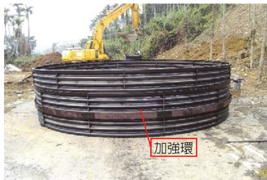
圖 4-19 型鋼加強環實體圖 steel hoop for structural reinforcement.
